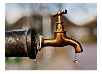
S A HOT WATER TAP DRIPS, water which was previously heated in a geyser leaves the geyser and is lost down the drain. But what is also lost is the heat energy held by that hot water. As the hot water drips away, leaving the geyser, new water will have to be continually added to the geyser and heated, thereby requiring an input of extra energy, usually electrical energy.
